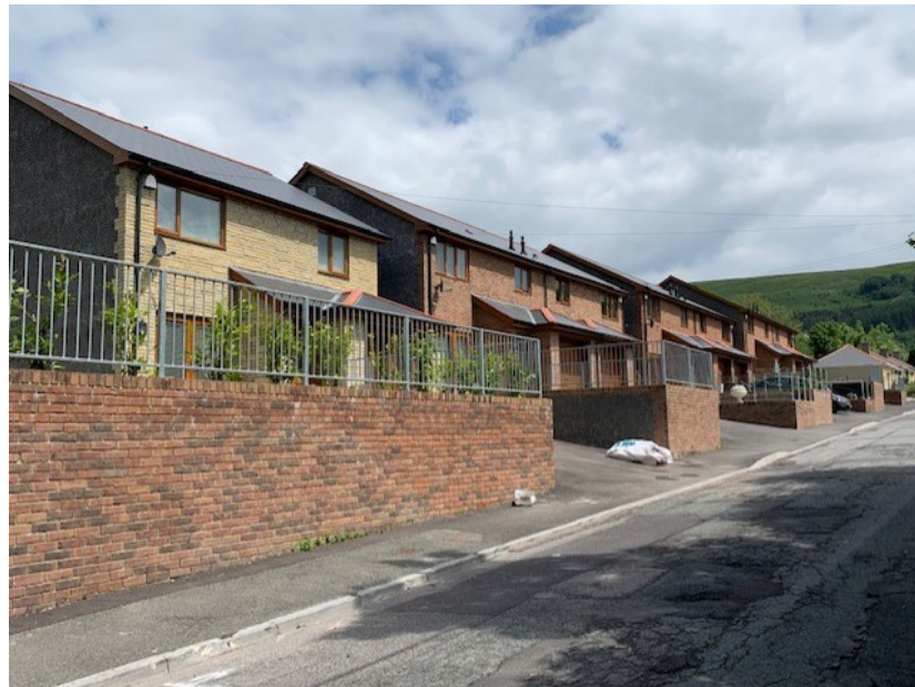
Photograph 5: showing brick walls and railings along the southern boundary fronting the properties. In two instances the railings have been replaced by glass screens.
