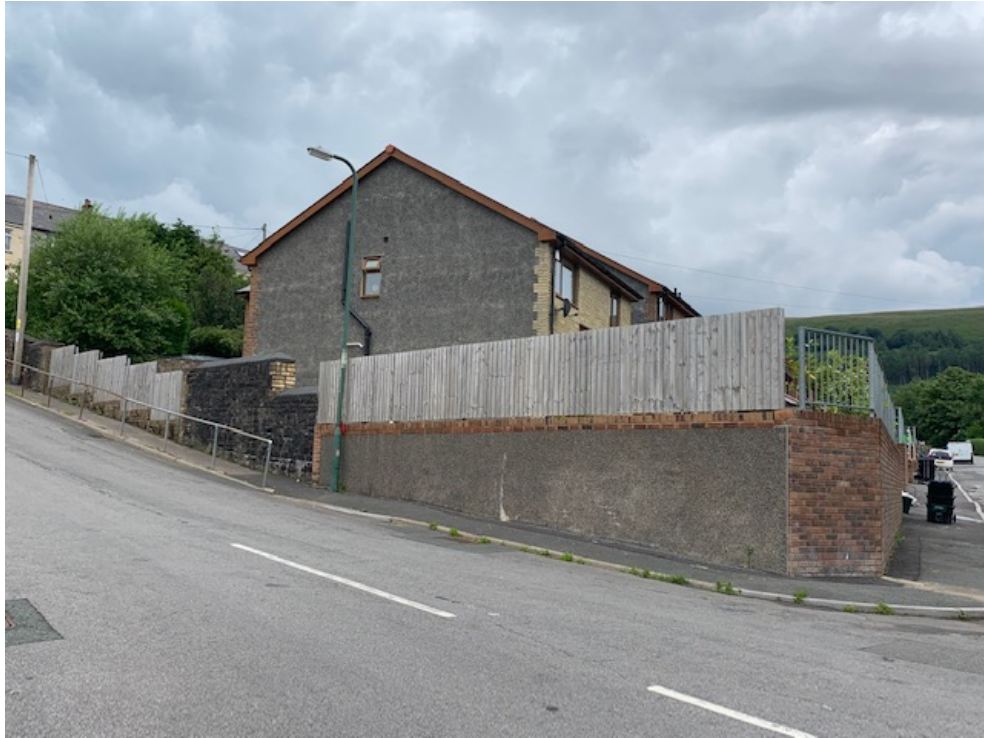
Photograph 9; Photograph of western boundary finishes where only a small section of the former school wall has been retained and the railings have been removed and the boundary has been demarcated by a rendered wall and close boarded fencing.
