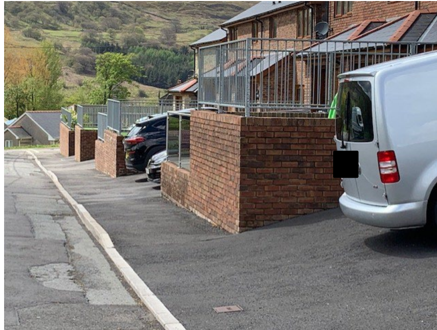
Photograph 23: Photograph showing frontage of site where vehicles would access/ egress over highway footpath in close proximity to high brick retaining walls.
