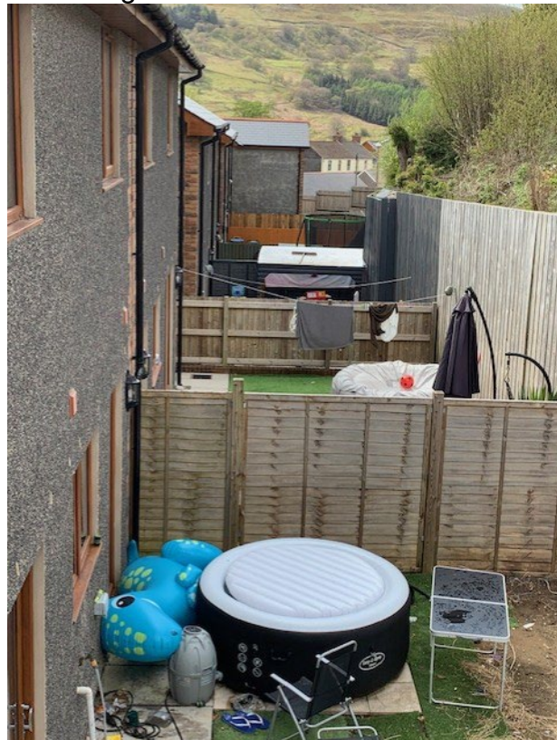
Photograph 8: showing the timber fence side boundaries between properties and a section of the new retaining wall constructed along part of the northern boundary with elevated garden areas relating to Gwent Terrace above.
