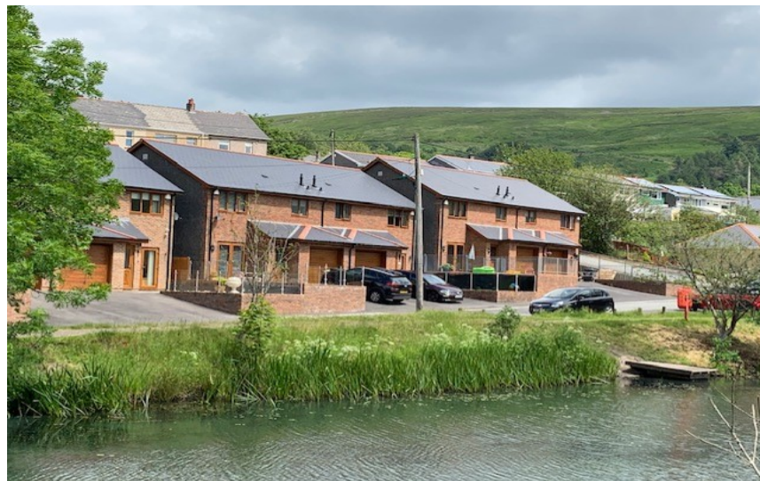
Photograph 3; showing front elevations of 3-7 Rhys yr Ysgol finished in brickwork
